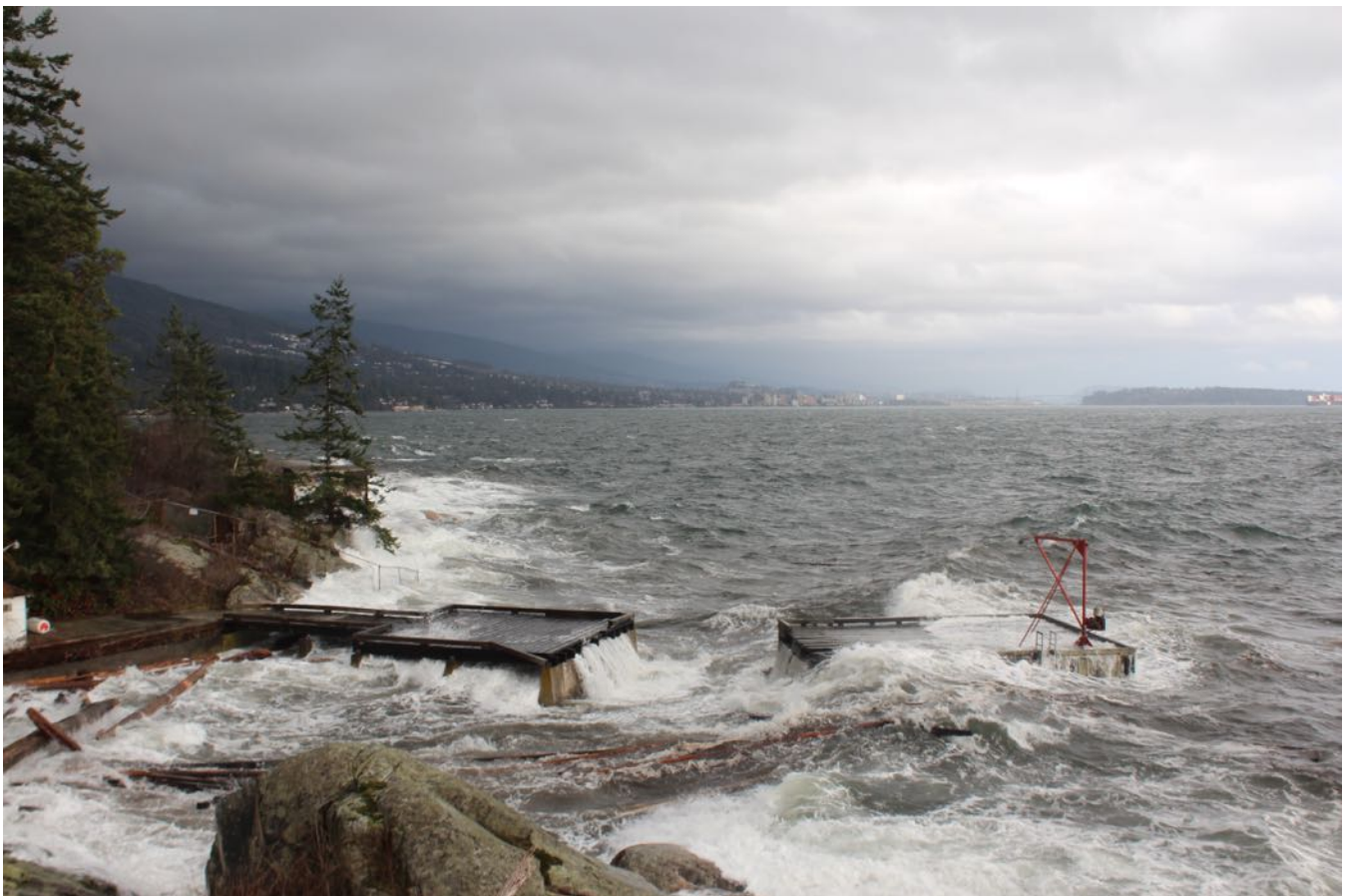
Broken dock at Point Atkinson Light Station. December 20, 2018
